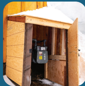
METER WITH SNOW SHELTER
